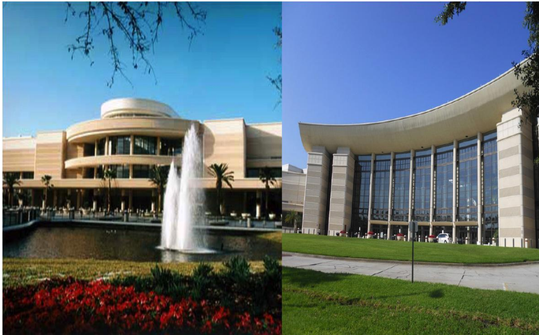
Wireless infrastructure deployed at the Orange County Convention Center & Peabody Hotel provided free Wi-Fi connectivity to all Cisco Live attendees in approximately 7 million square feet of floor area.
