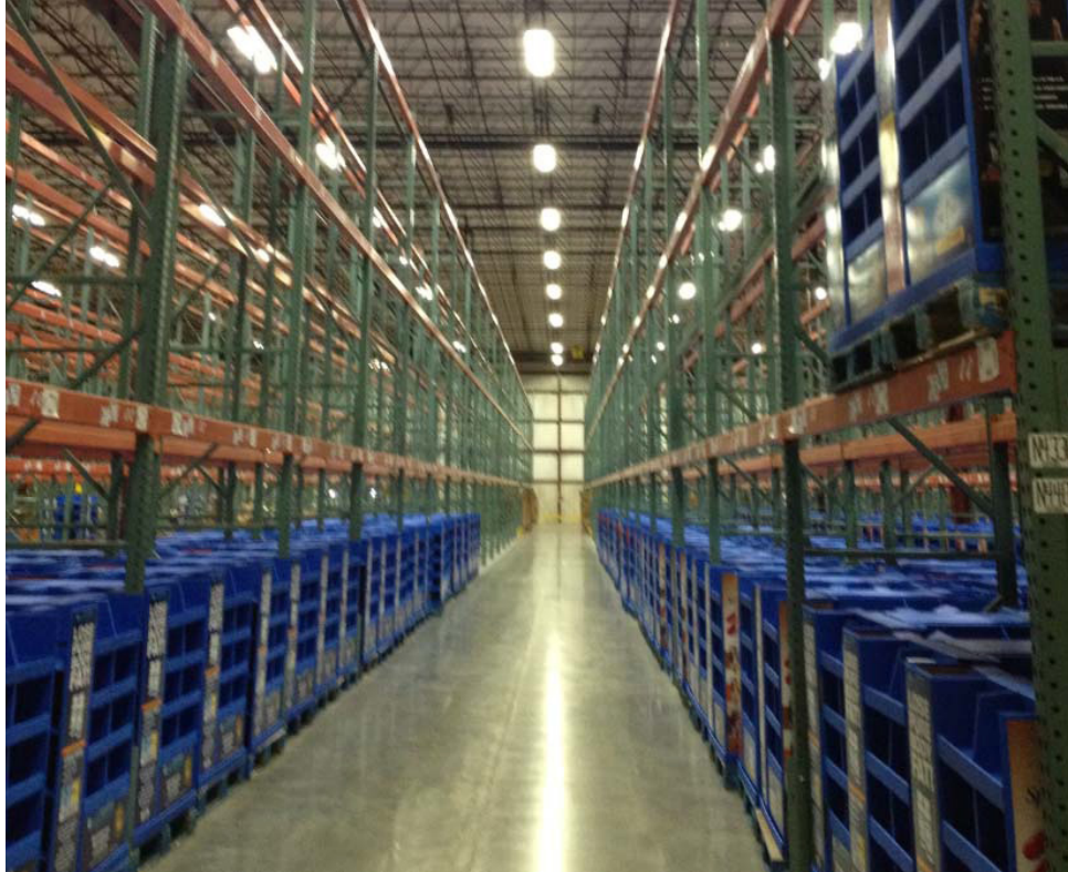
Figure 48 In areas where high amounts of metal is present, a site survey is required
