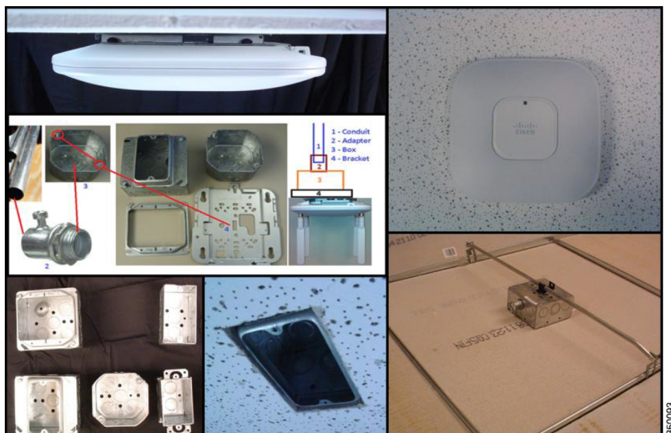
Figure 29 Mounting an AP onto an Electrical Conduit Box (ceiling T-Bar or conduit)
