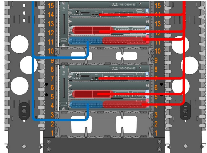
Figure 8 - Close-up view of resilient core routing
