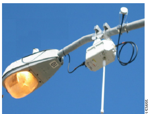
Figure 8-3 1500 Series Mesh AP Installation
